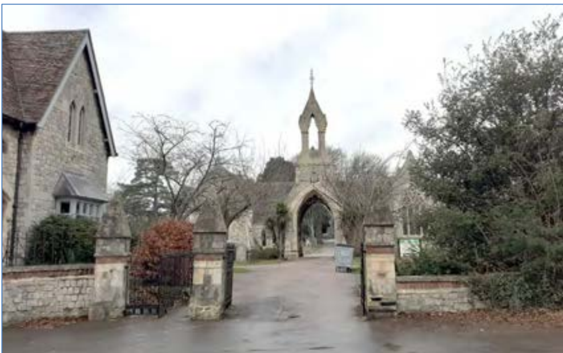
Fig. 12 Bell Road principal entrance to cemetery, wall and gatehouse
